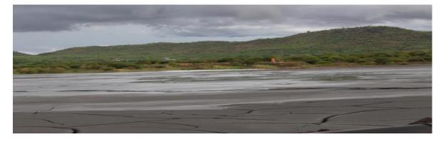
Tailings dam is typically an earth-fill embarkment dam used to store by products of Mining Operations after separating the ore from the Gangue.
